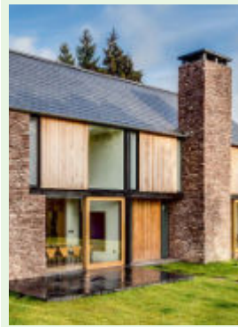
Stone bricks, larch cladding
