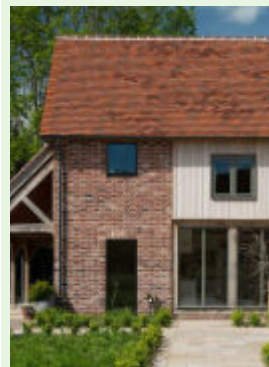
Brick, oak cladding, clay tiles
